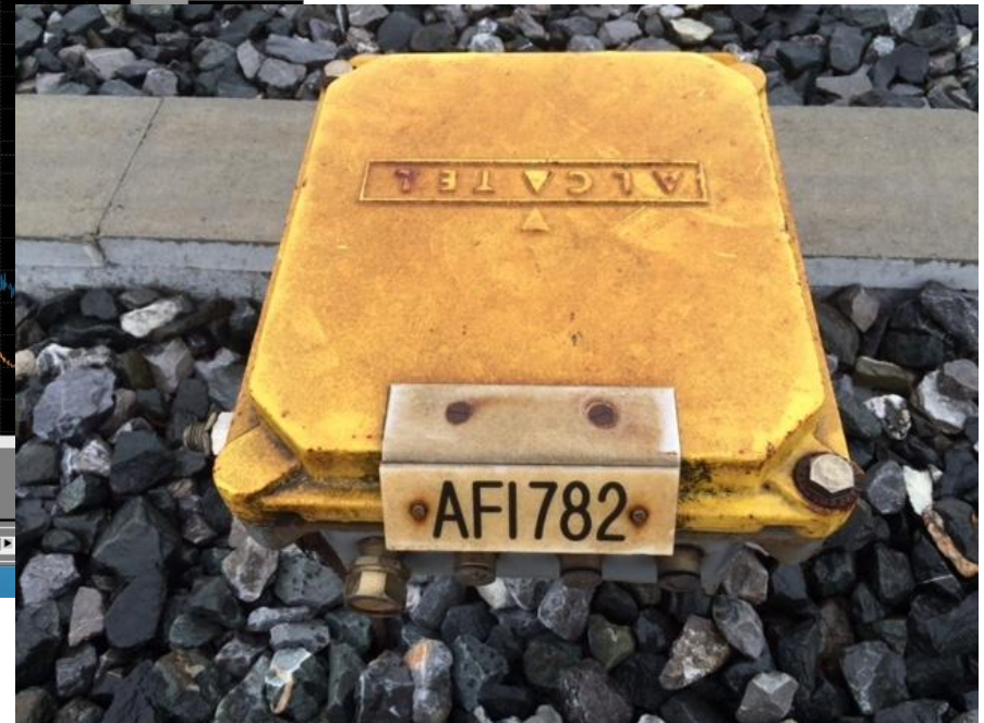
Traffic monitoring induction loop
